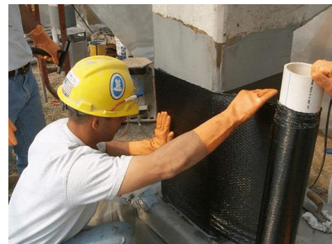
Fig. 2. Fragment of work on the reinforcement of columns with
