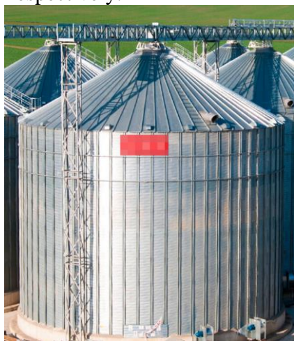
Fig. 1 – General view of grain drying complexes
